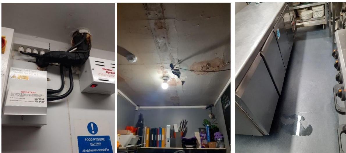
LEFT – DRIPPING WALK IN FREEZER PIPE. MIDDLE – DAMAGED OFFICE CEILING. RIGHT – POSSIBLE LEAKING FRIDGE.
