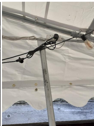
LEFT TO RIGHT - INDOOR FRIDGE LOCATED OUTDOORS AND INDOOR EXTENSION LEADS IN USE OUTDOORS.
