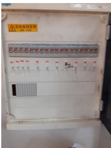
LEFT – HOLE IN THE TOP OF SWITCH CASING. MIDDLE – MISSING BLANK OR CIRCUIT BREAKER. BROKEN DISTRIBUTION BOARD CASING. RIGHT – INADEQUATELY INSULATED JOINED CABLES.
