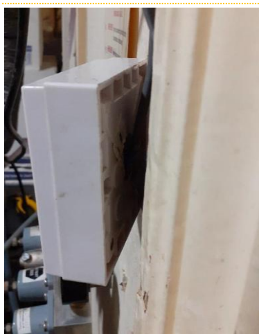
LEFT – LIGHT SWITCH INADEQUATELY SECURED TO THE WALL. MIDDLE – UNPROTECTED AND UNSUPPORTED CABLING RIGHT- BROKEN LIGHT SWITCH.
