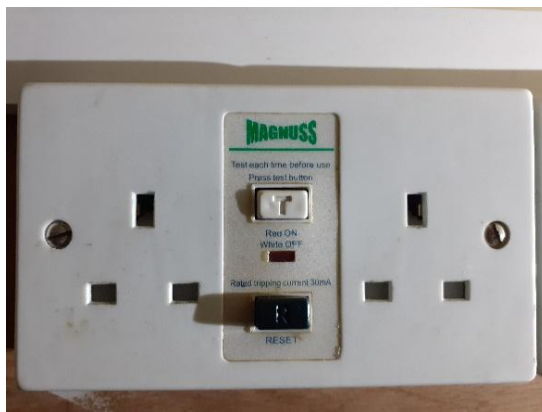
FIGURE 14 - ENTERTAINERS SOCKET WITH RCD PROTECTION IN A BRIDGEND NIGHTCLUB
