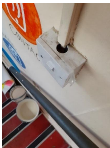
LEFT – HOLE IN THE TOP OF SWITCH CASING. MIDDLE – MISSING BLANK OR CIRCUIT BREAKER. BROKEN DISTRIBUTION BOARD CASING. RIGHT – INADEQUATELY INSULATED JOINED CABLES.
