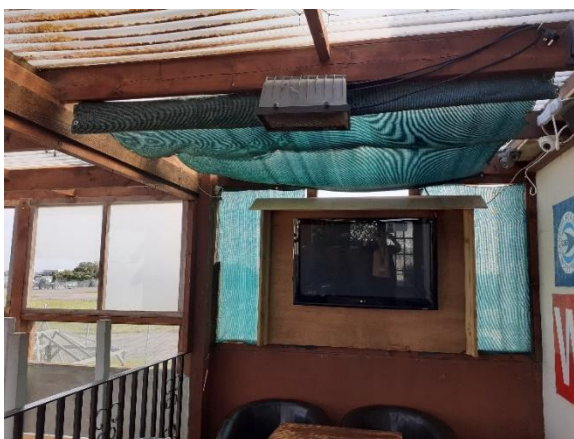
LEFT - INDOOR TELEVISION MOUNTED ON AN EXTERNAL WALL UNDER A CANOPY. RIGHT - INDOOR TELEVISION IN A PARTIALLY ENCLOSED AREA WITH AN INDOOR EXTENSION LEAD ON THE WALL TO THE UPPER RIGHT OF THE TELEVISION.
