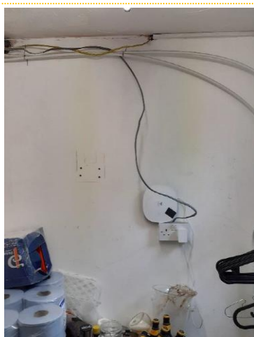
LEFT – LIGHT SWITCH INADEQUATELY SECURED TO THE WALL. MIDDLE – UNPROTECTED AND UNSUPPORTED CABLING RIGHT- BROKEN LIGHT SWITCH.
