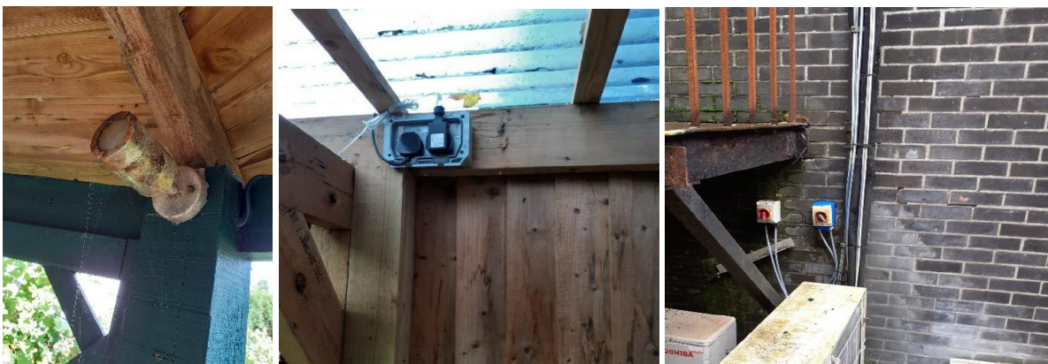
FIGURE 5 - PHOTOS FROM LEFT TO RIGHT SHOW A SIGNIFICANTLY CORRODED LIGHT FITTING, IP RATED SOCKET WITH BROKEN COVER AND A POORLY FITTING AND TAPED COVER TO A ROTARY ELECTRICAL ISOLATOR SWITCH.
