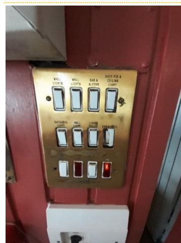
LEFT – LIGHT SWITCH INADEQUATELY SECURED TO THE WALL. MIDDLE – UNPROTECTED AND UNSUPPORTED CABLING RIGHT- BROKEN LIGHT SWITCH.
