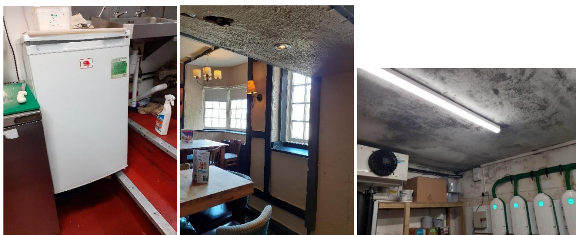
LEFT – INADEQUATELY SUPPORTED FRIDGE. MIDDLE – DAMAGE TO CEILING (ASBESTOS WITHIN VOID). RIGHT – MOULDY CELLAR.
