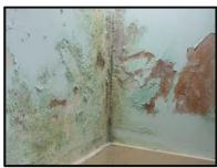
Rising damp will only occur on the ground floor. Signs of rising damp will usually include a damp stain along the base of a wall above the skirting board to a height of about 1.5m. Ground floor walls usually contain a damp proof course which is either built into or injected into the brickwork just above ground level. The purpose of the damp proof course is to stop water from the ground rising up through the brickwork. Rising damp can occur in the following situations –
