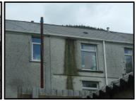
The first signs of penetrating damp will usually be damp stains appearing on an internal wall. Penetrating damp is caused by a specific defect with the property which is causing or allowing water to penetrate to internal surfaces. The most common causes of this kind of damp are detailed below.
