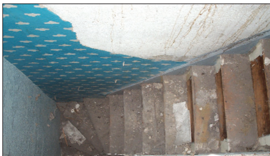
View of stairs from landing
